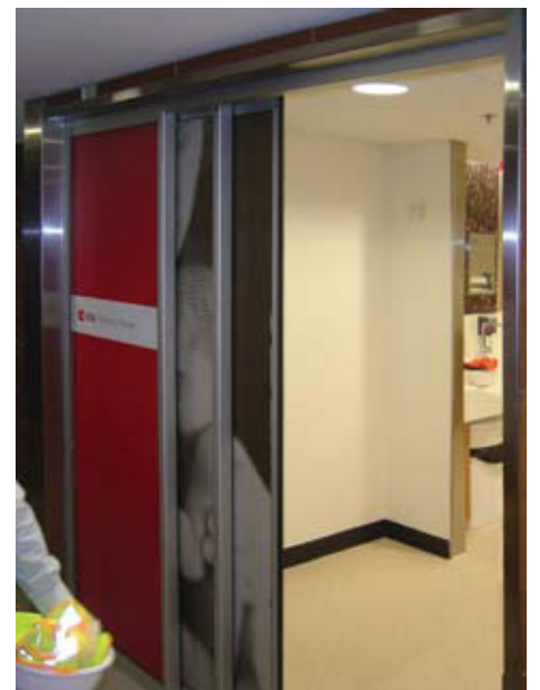
Confined doorway space, Maximum door opening using flush line glazing.
