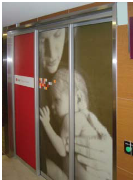
Confined doorway space, Maximum door opening using flush line glazing.
