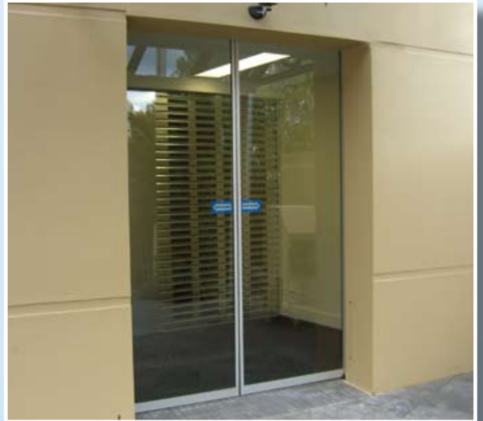
Designed for safer disabled access.
