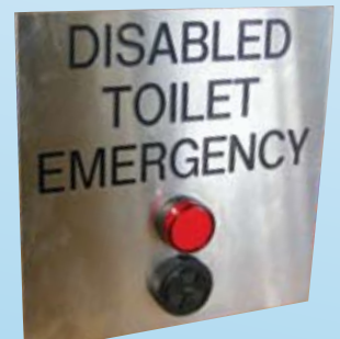
External strobe light and audible alarm.
